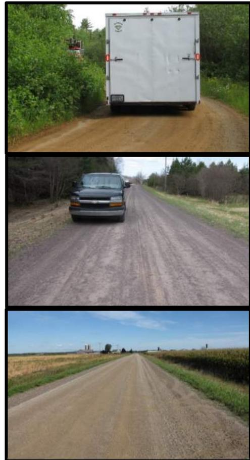
Figure 2: *Top*– Unpaved road with poor rating. *Middle*– Unpaved road with fair rating. *Bottom*– Unpaved road with good rating.
