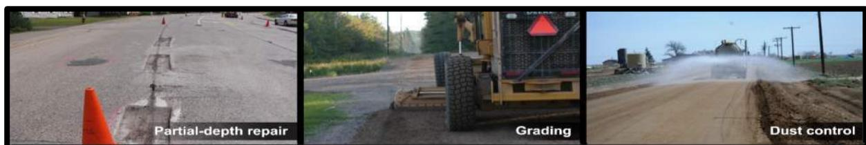
Figure 6: Examples of capital preventive maintenance treatments, cont’d—(from left) concrete road prepared for partial-depth repair, gravel road undergoing maintenance grading, and gravel road receiving dust control application (dust control photo courtesy of Weld County, Colorado, weldco.gov)
