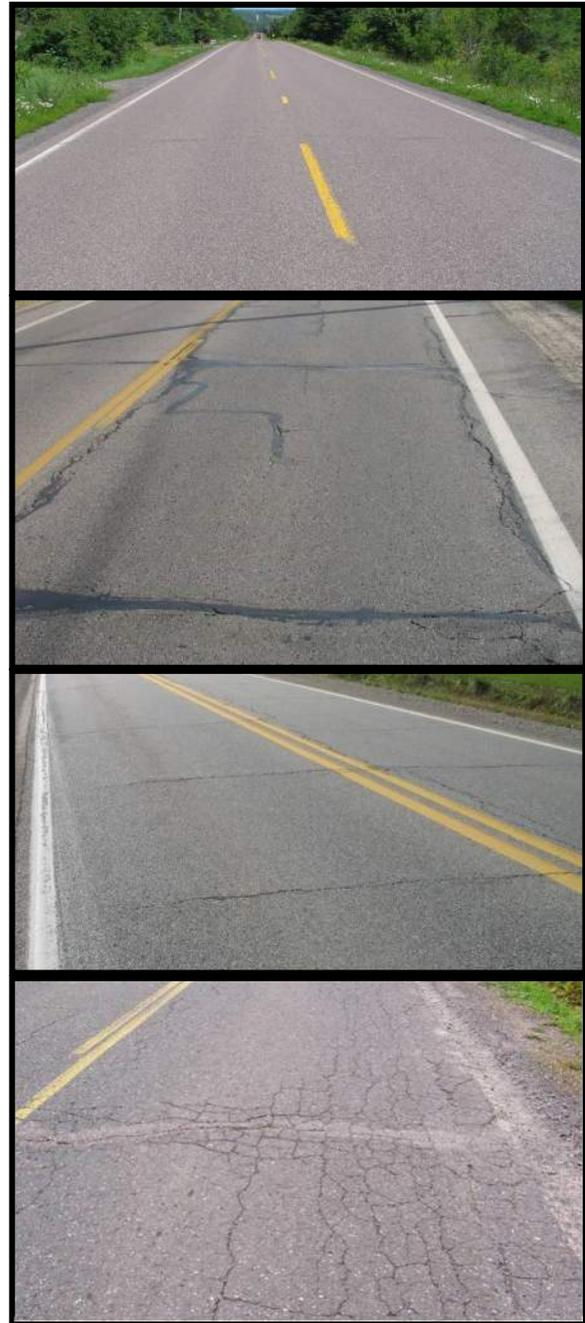
Figure 1: *Top image, right*– PASER 8 road that is considered “good” by the TAMC exhibit only minor defects. *Second image, right*– PASER 5 road that is considered “fair” by the TAMC. Exhibiting structural soundness but could benefit from CPM. *Third image, right*– PASER 6 road that is considered “fair” by the TAMC. *Bottom image, right*– PASER 2 road that is considered “poor” by the TAMC exhibiting significant structural distress.
